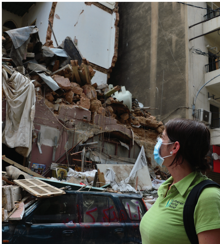
A Lutheran World Relief team member surveys damage in Beirut caused by a blast that ripped through the city's port area on August 4.
