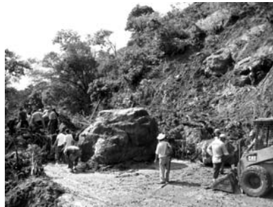
Members of the community of San Pedro Nonualco survey a road damaged by a landslide. Photo courtesy of FUNDE.
